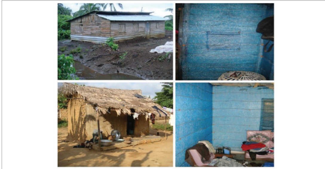
Figure 6: Durable linings (B) installed in traditional houses in rural Equatorial Guinea (A) and in Ghana (C, D) 47 .
